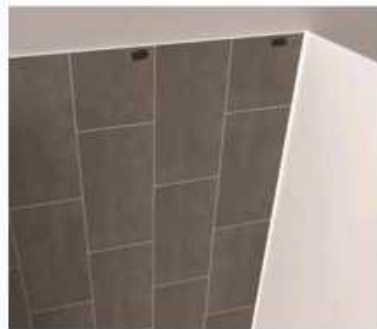
5、敲打使墙板紧凑 5. Tap to compact the wall panels
