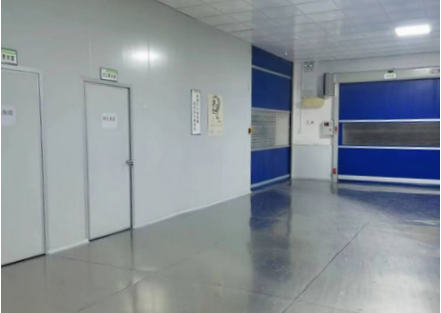
Radar sensor automatic doors 雷达感应自动门
