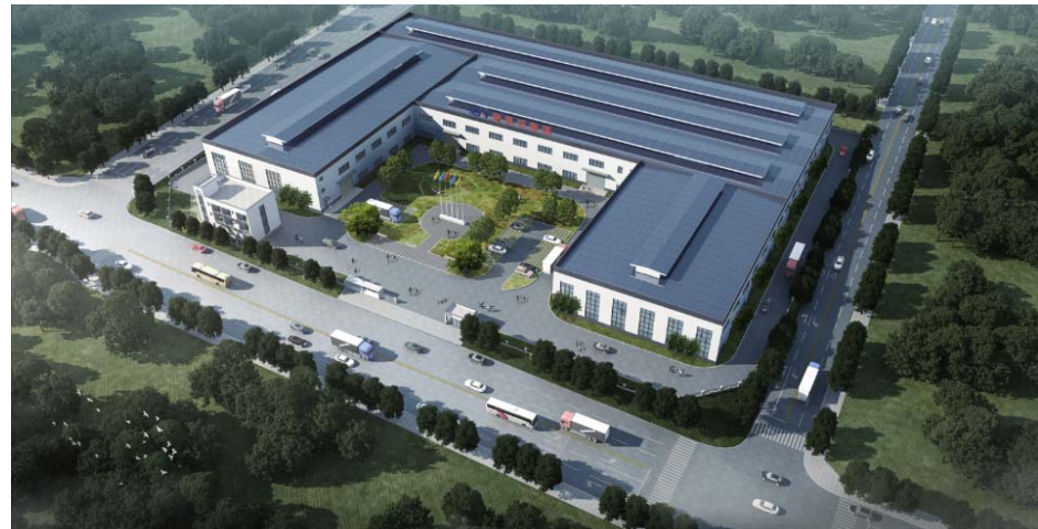
RST Casting Factory
