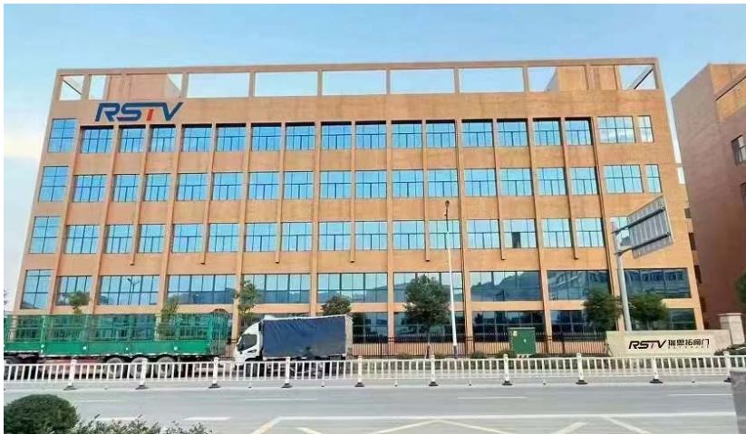
RST Headquarters (2 Buildings)
