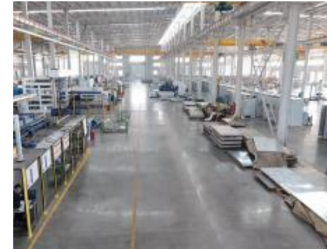
壳体车间 Casing workshop Atelier Shell
