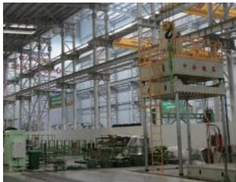
220KV线圈绕制 220KV coil winding Bobine 220kV enroulée
