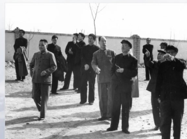
三线建设期间 由上海搬迁至宁夏 In 1965, our company was moved from Shanghai to Ningxia during the period of the Third Front Movement.
