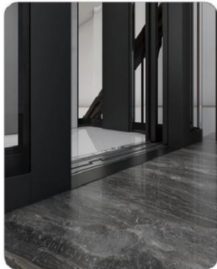
Achieving perfection in the unseen details A 10mm threshold gap is not only a precise control within industry standards,but also our persistent pursuit of safety and smoothness. Wheelchairs and strollers pass through smoothly without jerks,high heels navigate freely without restriction,and phones are prevented from falling.This perfectly measured spacing allows stability and fluidity to coexist in perfect balance.
