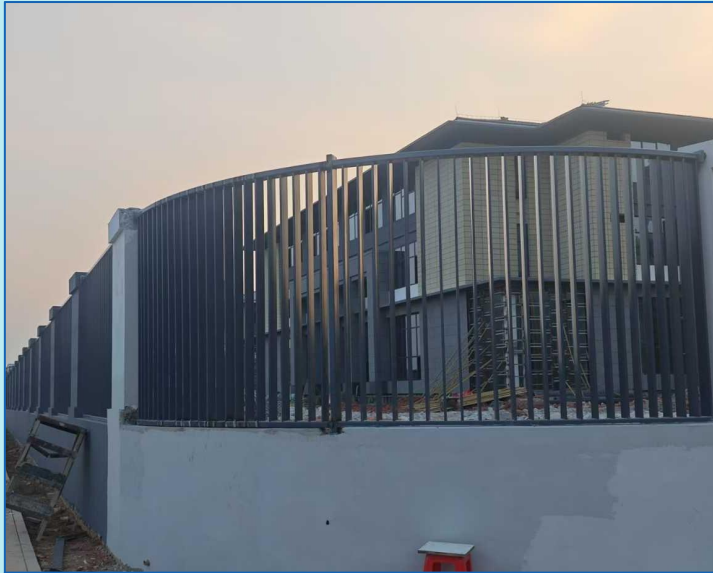
Y043 Villa Perimeter Guardrail
