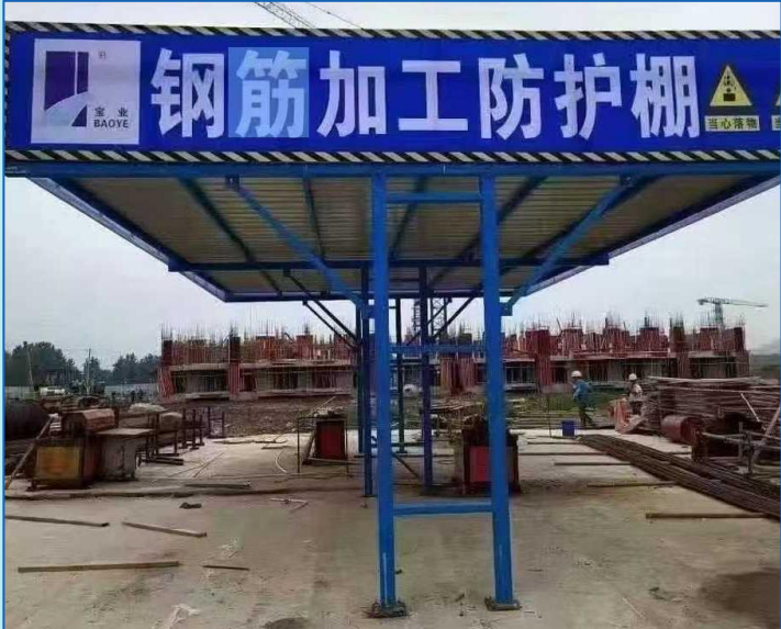
Y087 Twin-column Rebar Shelter
