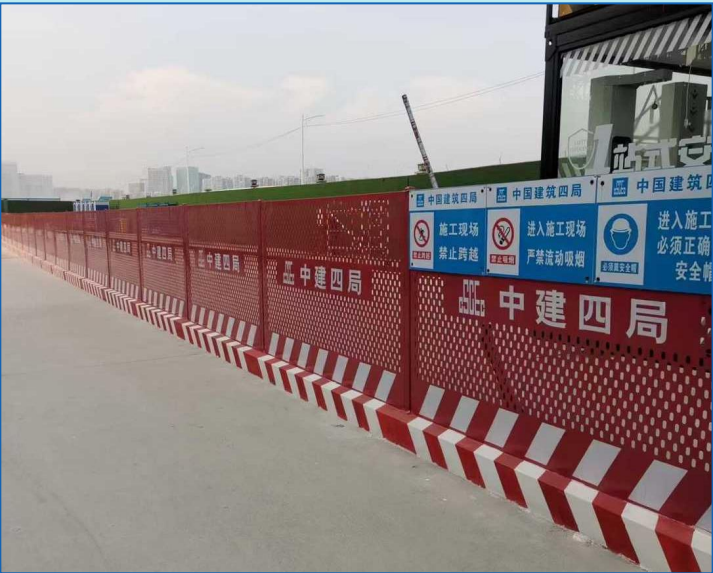
Y083 Perforated Excavation Guardrail
