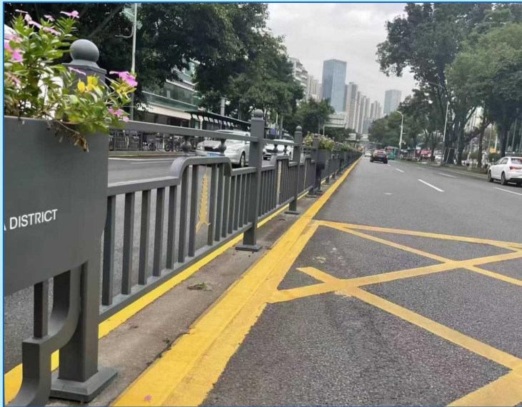
T004 Planter-box Cultural Guardrail
