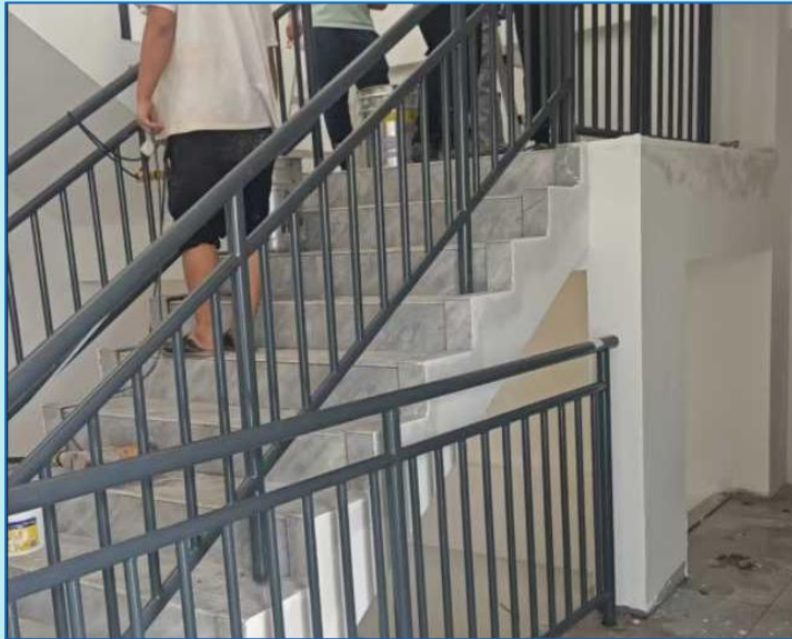
Y061 Zinc-steel Stair Guardrail
