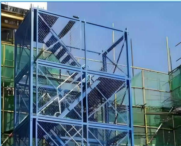
Y092 Stair Cage
