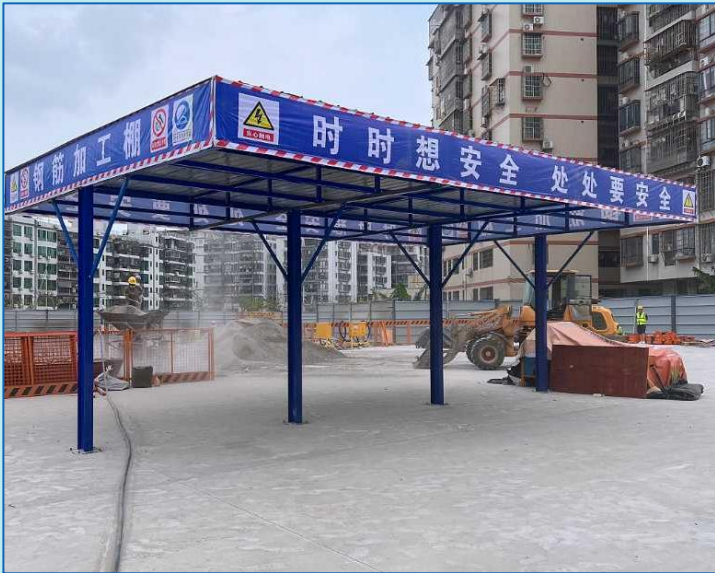
Y086 Rebar Processing Shelter
