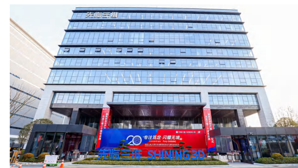
Building D: R&D Center, Accuracy Lab, Production Base
