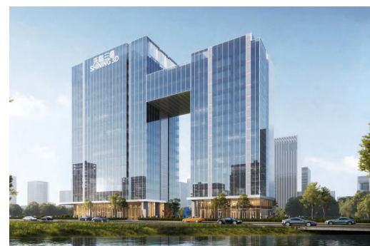
Building C: Software Development and Headquarters Base (Under Construction)
