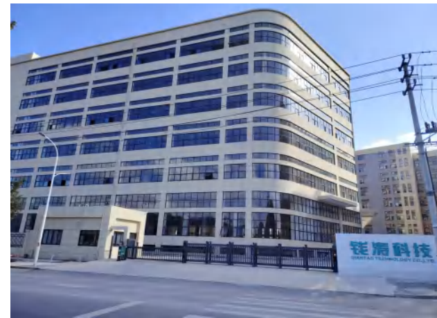
New factory under construction
