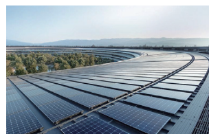
Factory Solar System
