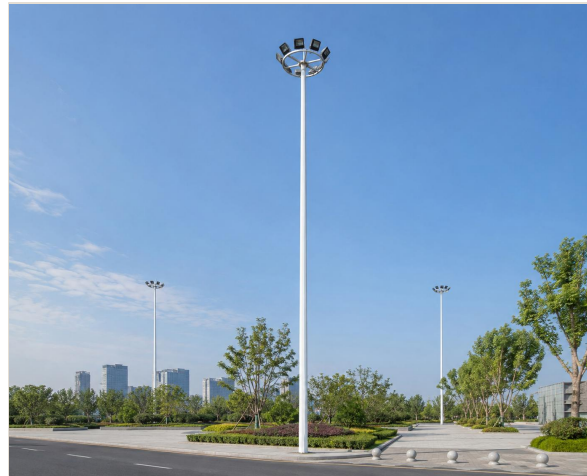
Cluster Head Area Mast
