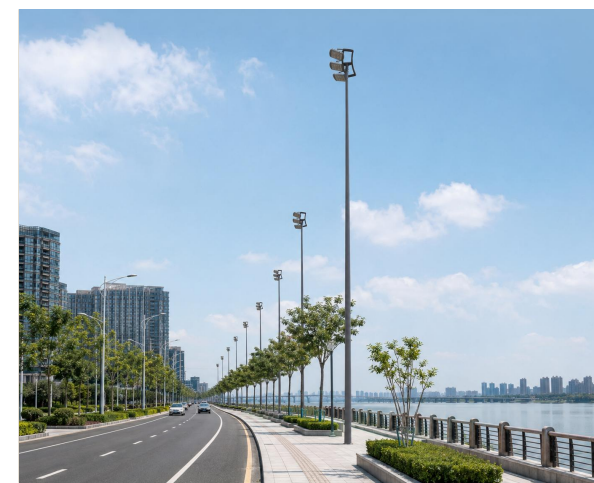
Stadium Cluster High Mast
