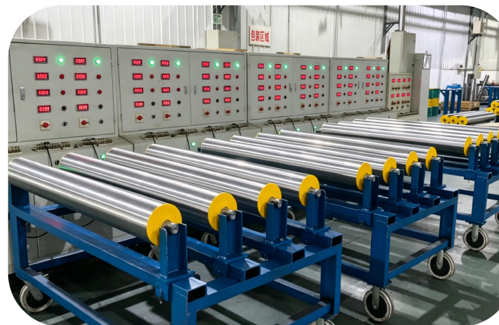
Voltage & Current inspection
