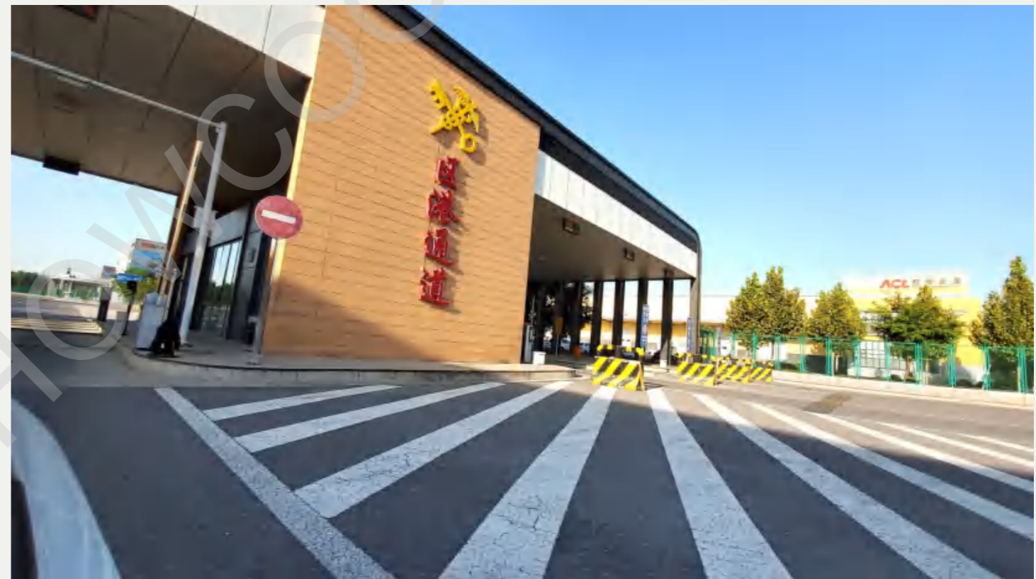
Customs inspection cold storage project of Beijing Shunyi Airport Logistics Park
