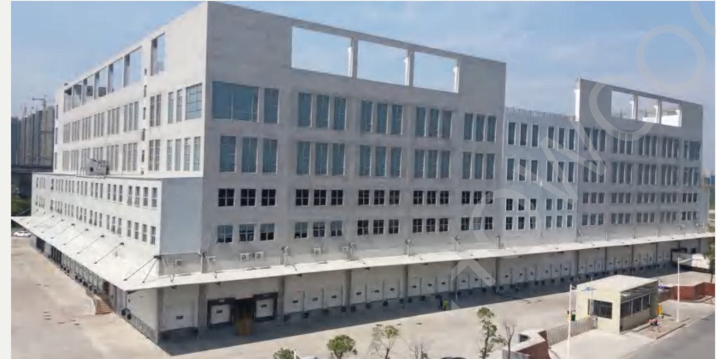
20000 tons cold chain logistics cold storage project
