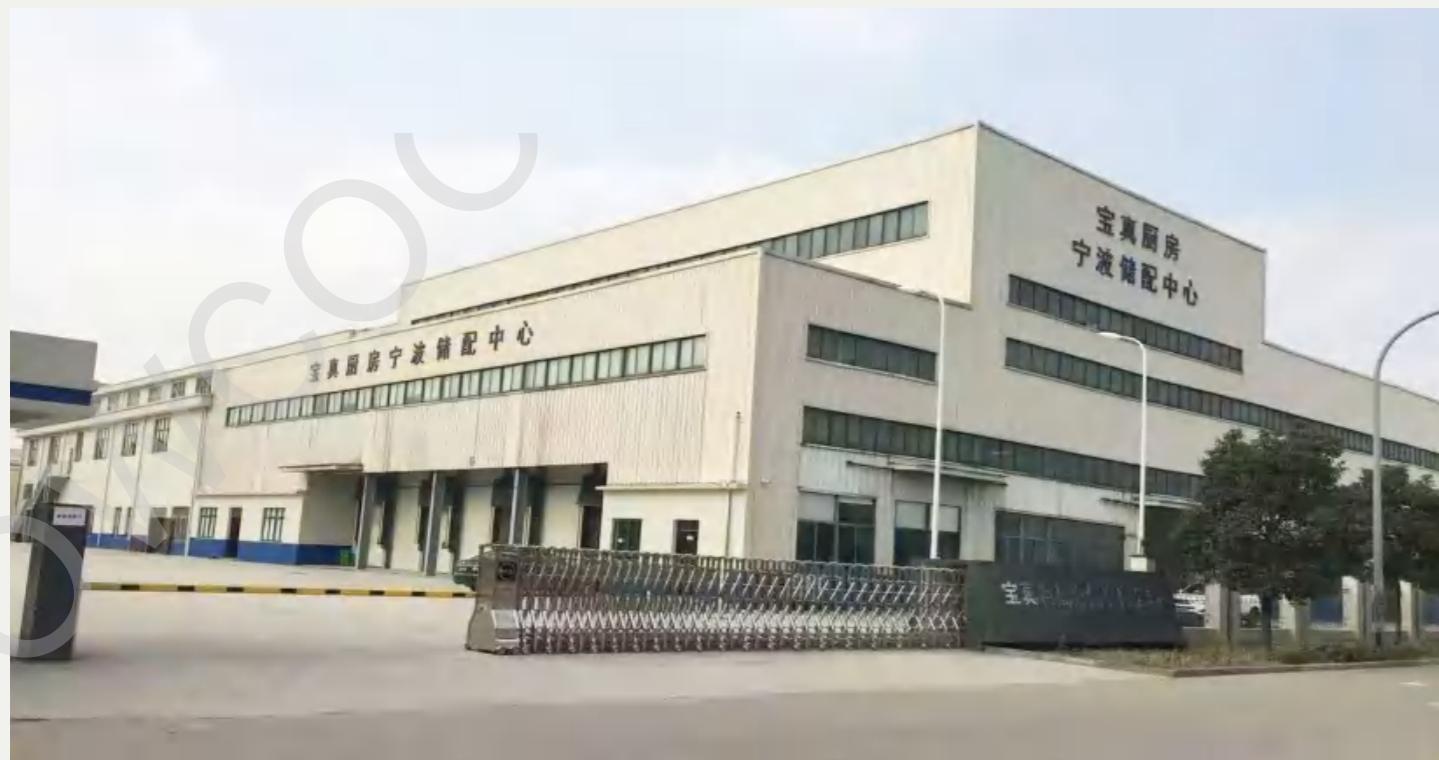
Cold storage project of central kitchen
