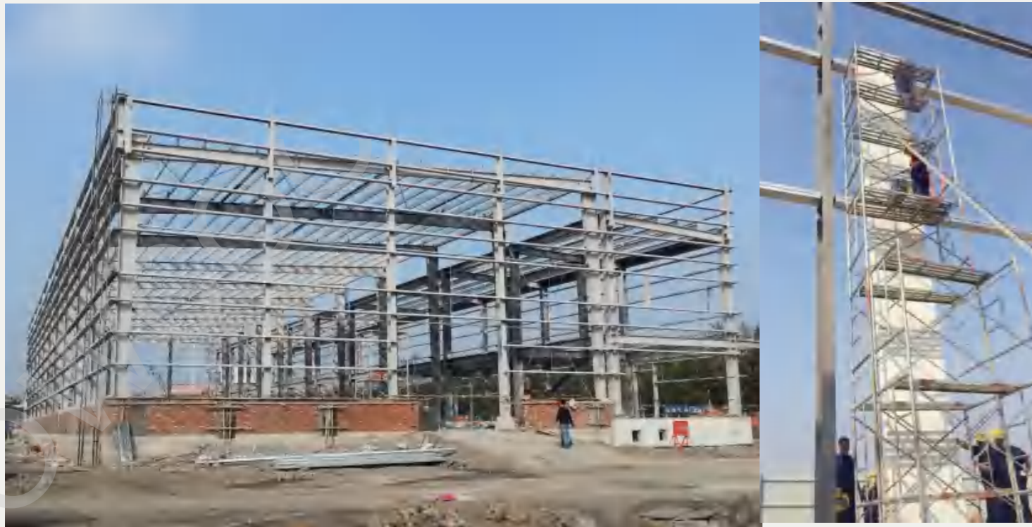
Main body of steel structure
