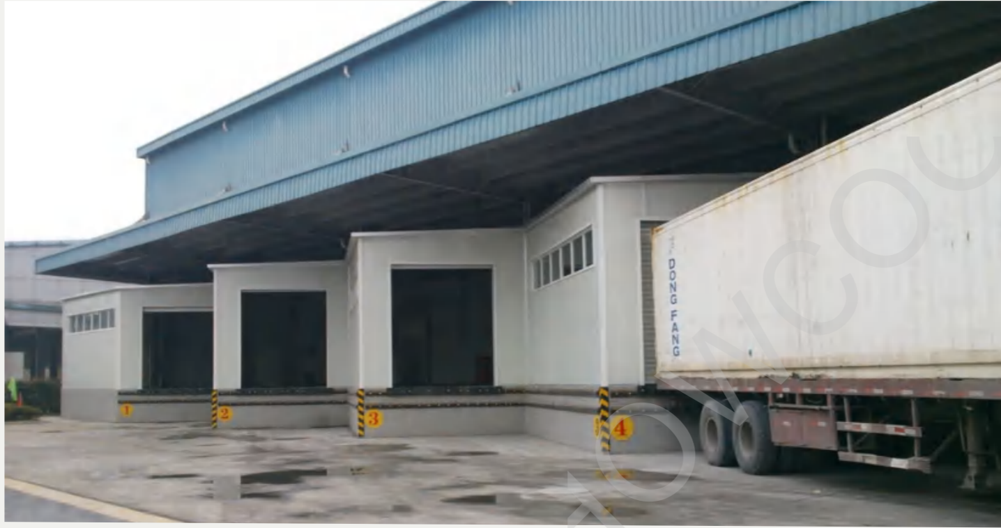
E-Commerce Distribution Center At Beijing
