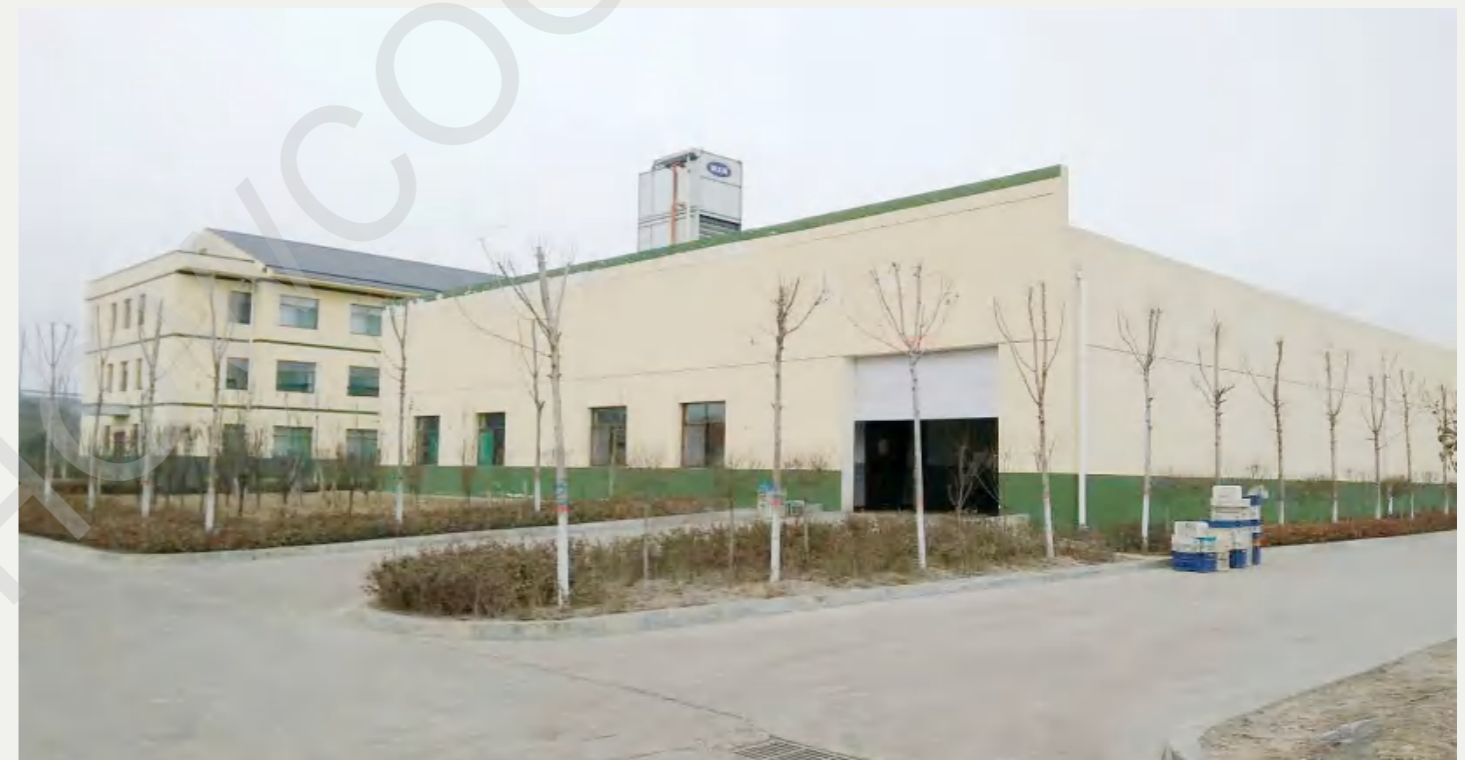
Cold storage of agricultural products logistics center
