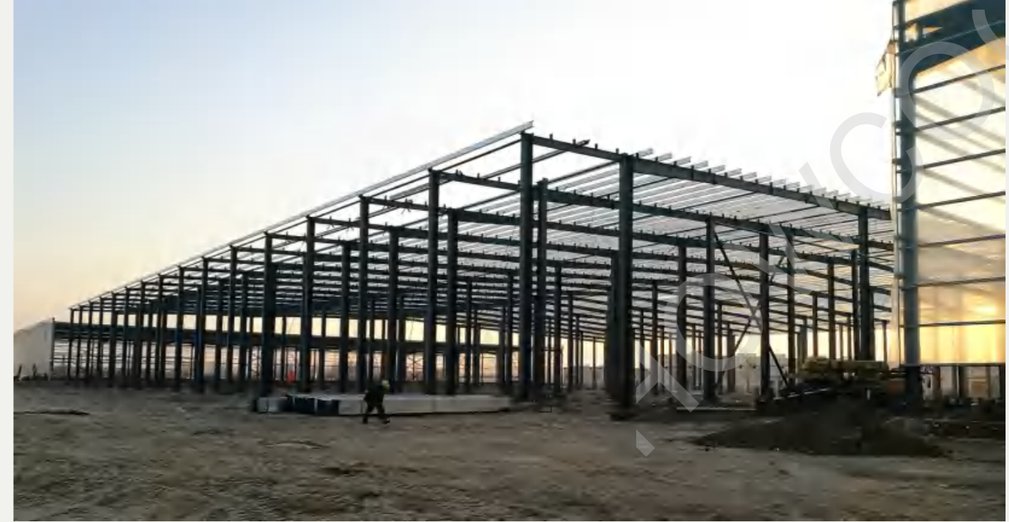
Main structure of large steel cold storage
