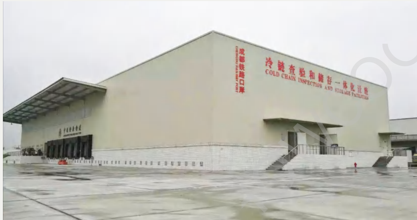
5000 ton cold storage project at railway port
