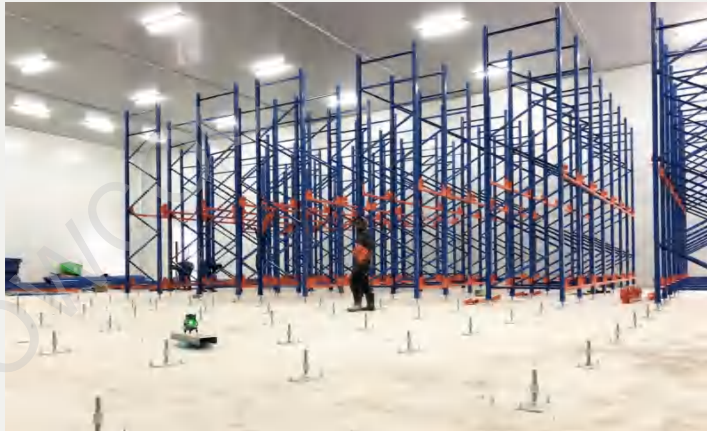
Shuttle Rack Installation
