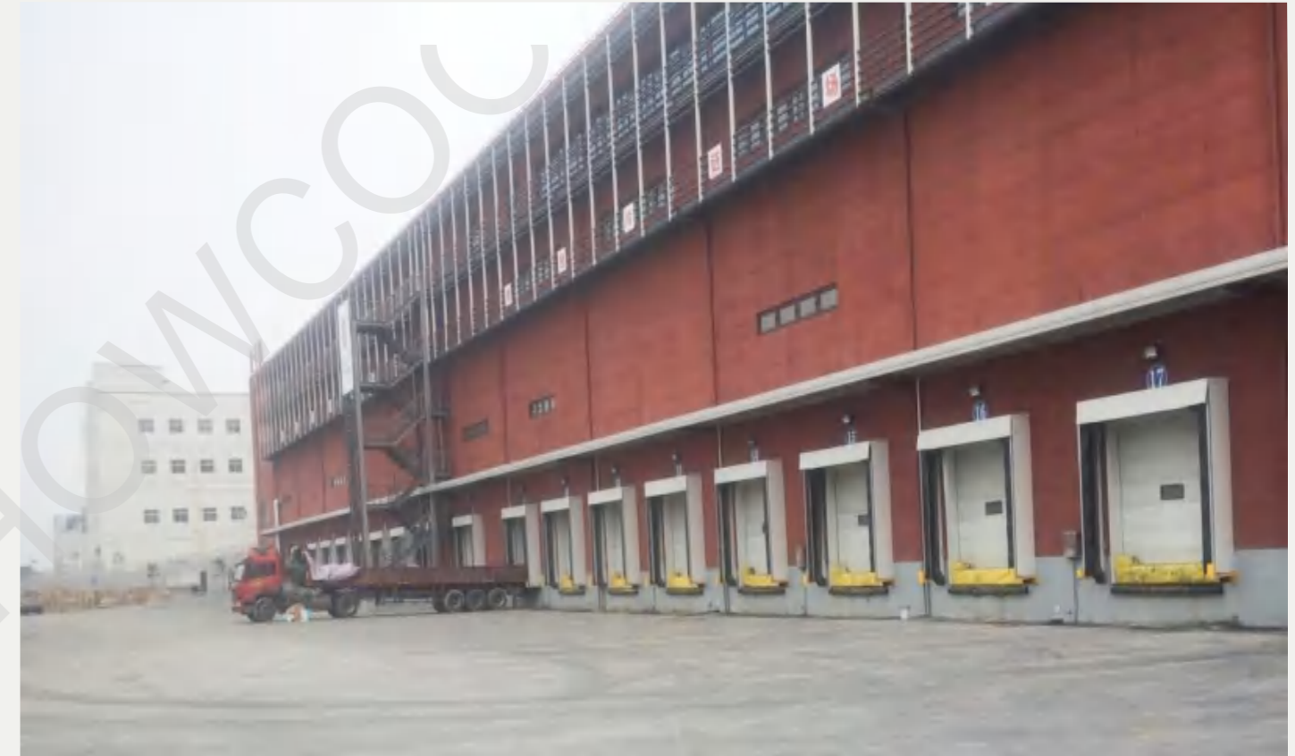
logistics Cold Store Project At Shanghai
