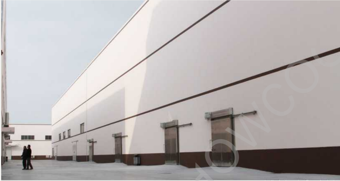
50000 cubic meters of e-commerce food cold storage
