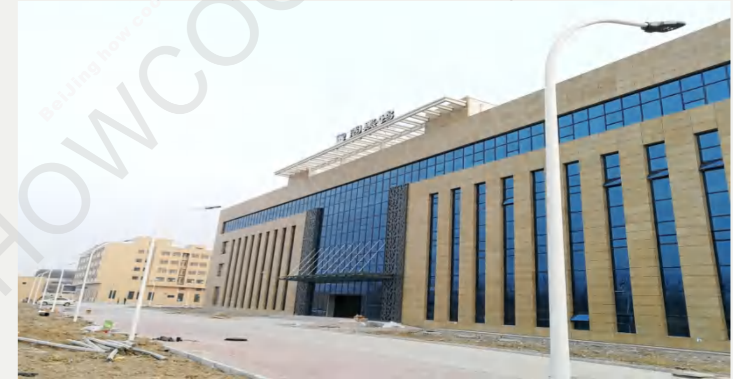
Cold storage project of food processing plant
