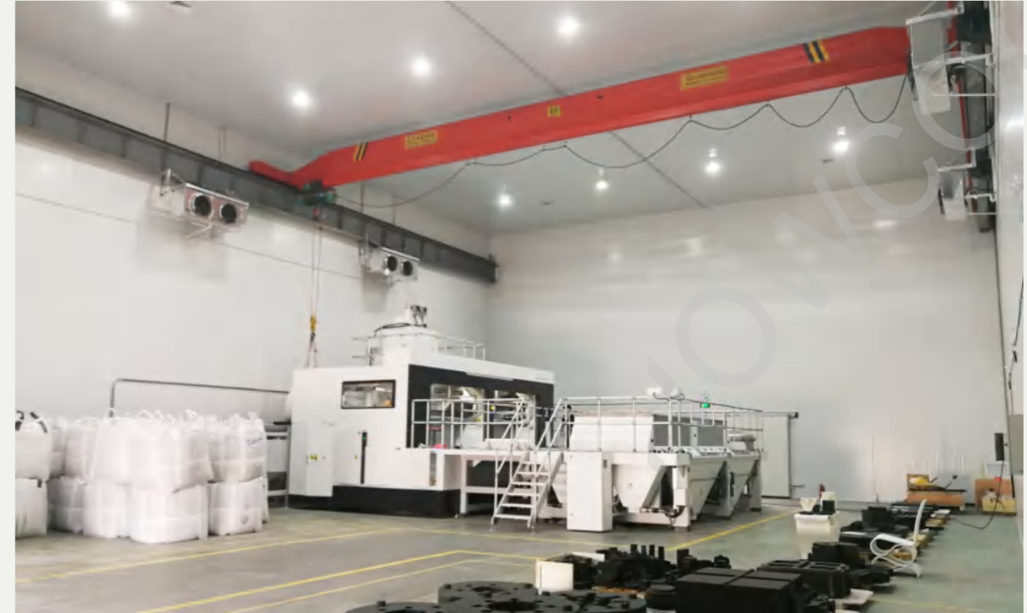
National intelligent casting 3D printing center
