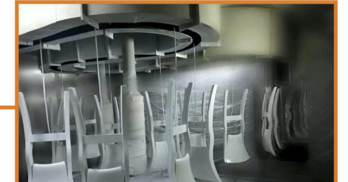
静电喷房 Electrostatic Spraying Room
