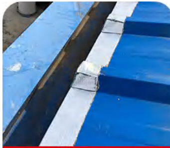
Color steel tile repair
