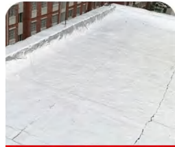
Bungalow roof waterproofing
