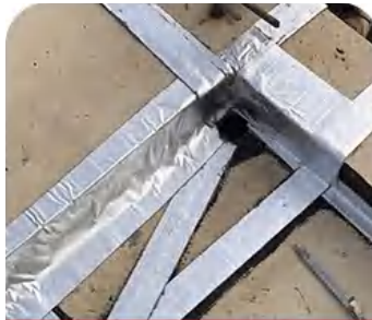
Crack repair
