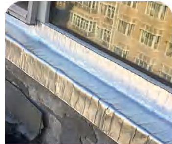
Window sill seam waterproof
