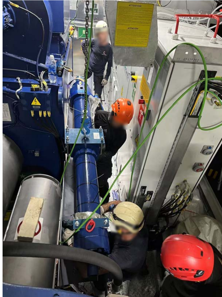
Pitch Cylinder Replacement
