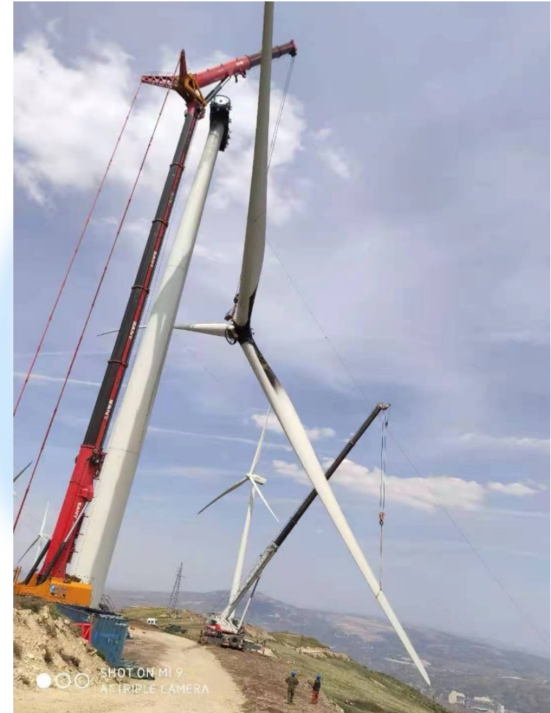
Turbine Dismantling
