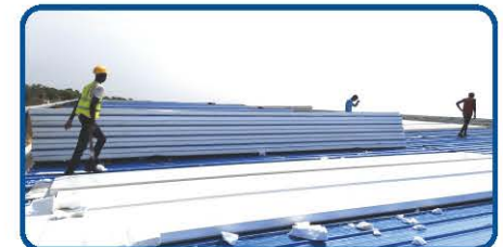
屋顶瓦的安装 install the roof panels
