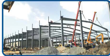
梁柱吊装 Install the columns & beams by crane
