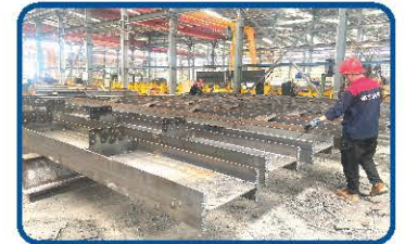
打磨清渣 Grinding and slag removal
