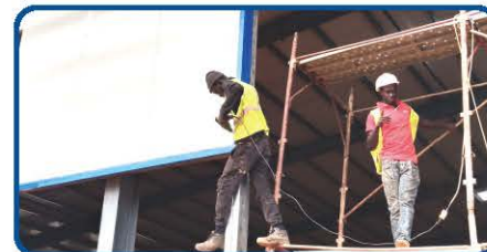
各包边的安装 install the flashing sheets
