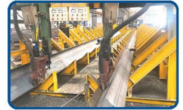
埋弧焊 Submerged arc welding
