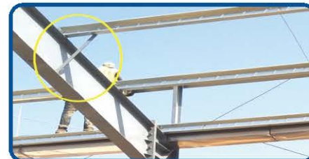
檩条隅撑 install the purlin bracing
