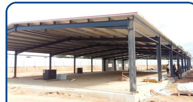
钢结构餐厅 steel structure canteen
