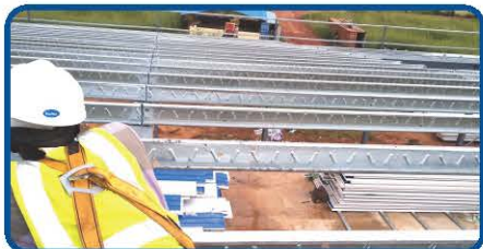
屋面檩条 install the roof purlin
