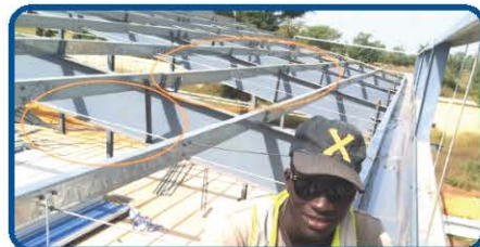
檩条拉杆 install the purlin rod
