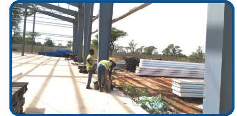
墙面檩条 Install the wall purlins
