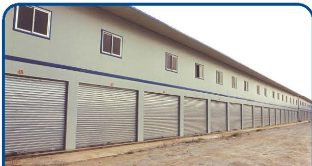
钢结构商铺 prefabricated store
