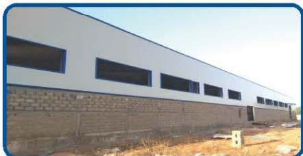
墙板的安装 Install the wall panels
