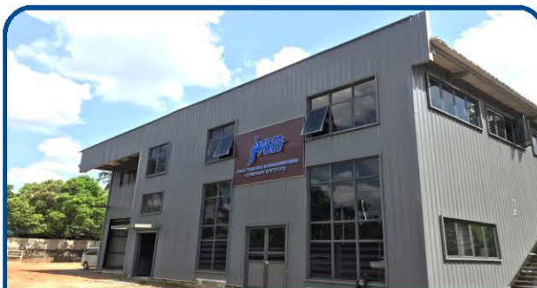
钢结构厂房 steel structure workshop
