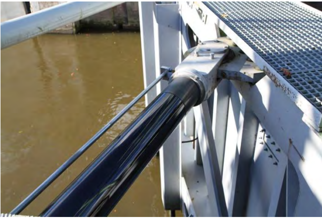
船闸液压启闭机陶瓷活塞杆 Ceramic piston rod of ship lock hydraulic hoist
