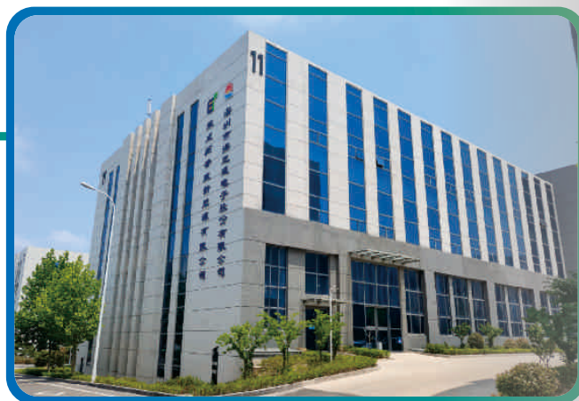
Shandong R&D Engineering Technology Manufacturing Base
