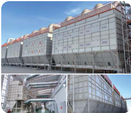
双级脉冲布袋除尘器 Dual Stage Pulse Dust Precipitator
