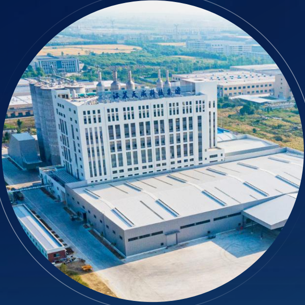
Exhaust Gas Treatment in Feed Production
