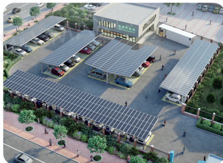
PV Charging Carport With Storage
