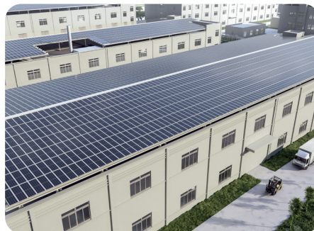
Flat-to-pitched Roof Conversion
