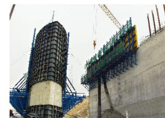
Project name: Qingshan Reservoir, Dandong, Liaoning Province Contractor: China Water Resources and Hydropower, No. 6 Engineering Co., Ltd. Products utilized: CB-240(Diagonal Brace Type)
