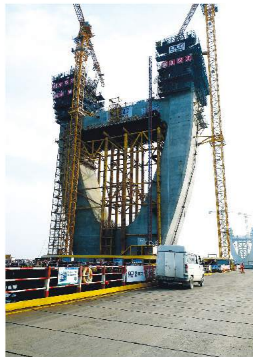
Project name: Section 1, 2, 3 of the main channel of Zhoushan Port, Ningbo Contractor: Zhejiang Jiaogong Group Co., Ltd. CSCEC China Communications Road and Bridge Construction Co., Ltd. Products utilized: ACS, HCB-100 (Separate Truss Type)
