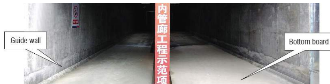
Site preparation before installation
