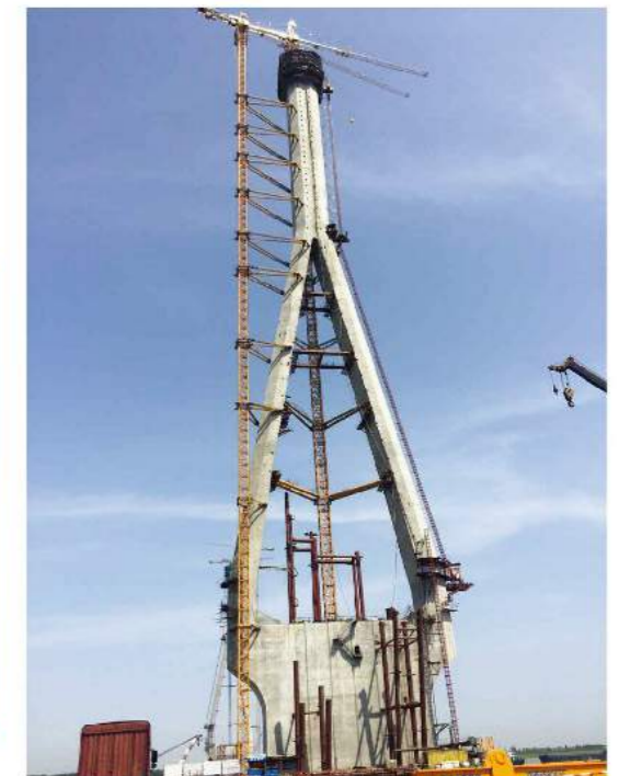
Project name: Wangdong Yangtze River Highway Bridge Contractor: South China Engineering Co., Ltd. of China Communications Road and Bridge Construction Co., Ltd. Products utilized: ACS, HCB-100 (Composite Truss Type)
