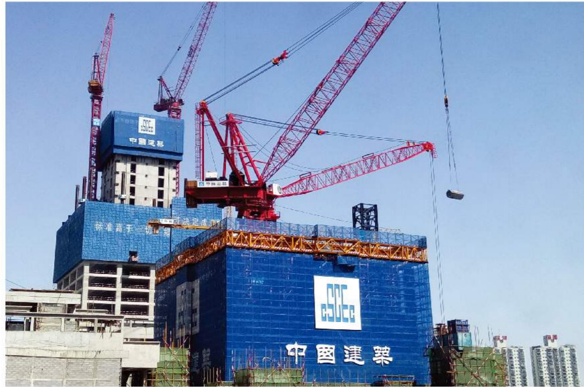
Project name: Shenyang Baoneng Global Financial Center T1、T2 Contractor: CSCEC, Third Bureau Products utilized: ACS, HCB-100 (Separate Truss Type)
