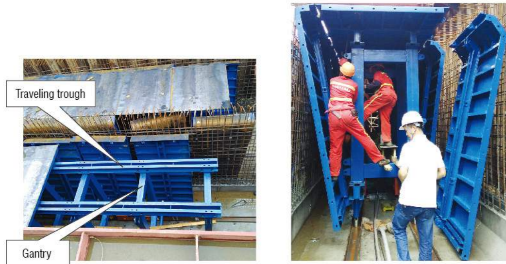
Installation of top stringer and formwork
