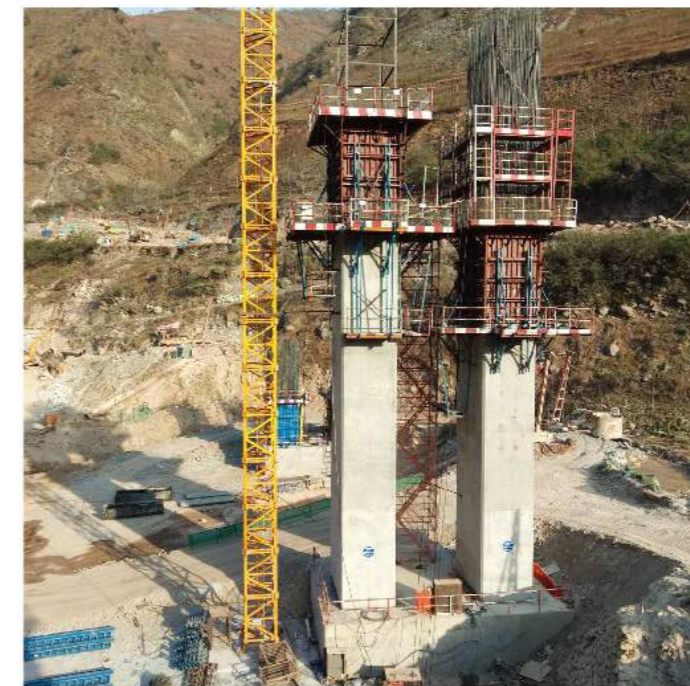
Project name: Wusi River Bridge Contractor: Sichuan Highway and Bridge Construction Group Co., Ltd. Products utilized: CB-240(Diagonal Brace Type)
