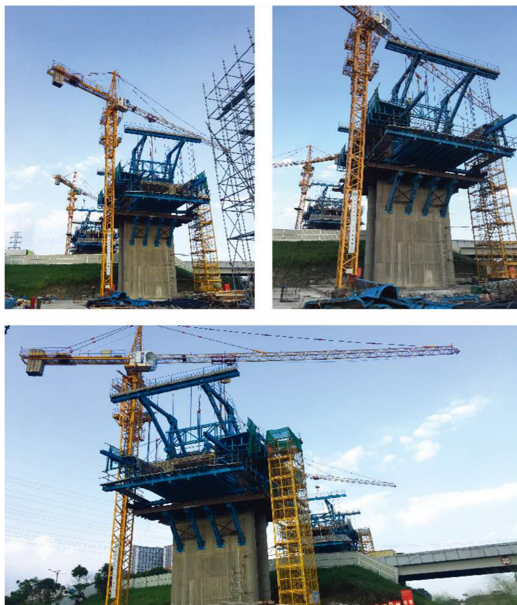
Project name: Jakarta-Bandung High Speed Railway Contractor: High Speed Railway Contractor Consortium- Project Team China Railway Group Limited Products Utilized: Cantilever Forming Traveler
