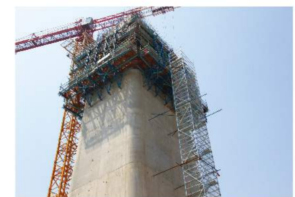
Project name: Hutong Yangtze River Bridge Pier Contractor: China Railway Bridge Group Fourth Engineering Co., Ltd. Products utilized: CB-240 (Truss Type)
