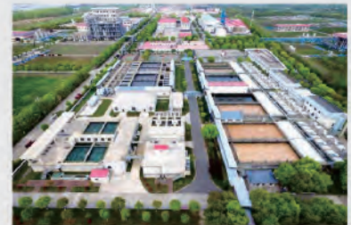
Wastewater treatment plant of Anhui Guoxing Biochemical Co., Ltd
