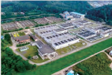
Phase II of Hengling Water Purification Plant in Shenzhen
