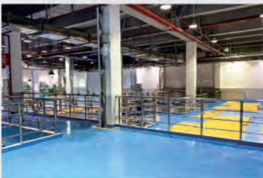
Chengdu Dougou River Wastewater Treatment Plant II
