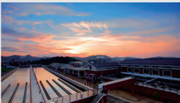
Zhoushan City Water Supply Co., Ltd Scal: 700,000m 3 /d
