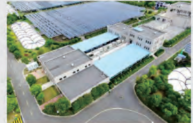
Hefei Wangxiaoying Wastewater Treatment Plant
