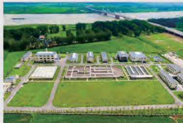
Wuhe County Chengnan Wastewater Treatment Plant
