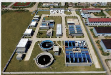
Hexian Huaqi Chemical Wastewater Treatment Co., Ltd
