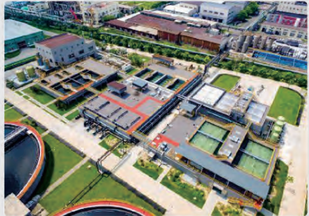
Expansion and upgrade of Jiaxing port area's industrial wastewater plant (renovation)
