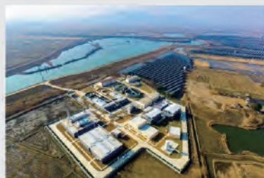
Wastewater Treatment Plant, South Hanshan Econ. Dev. Zone
