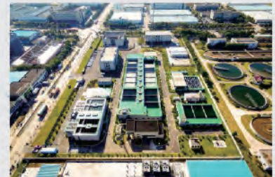
Ma'anshan Southern Town Wastewater Treatment Plant
