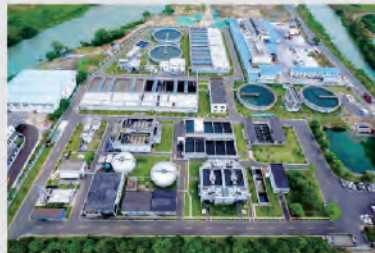
Yixing Dingshu Wastewater Treatment Plant
