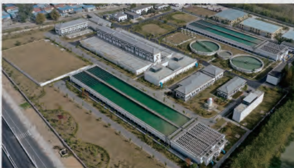
Huai'an Water Supply Co., Ltd Scal: 690,000m 3 /d
