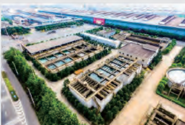
Changzhou Zhongtian Steel Wastewater Treatment Plant
